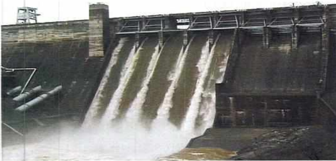
Fig. 7.8 Dam water generates electricity
