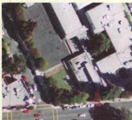
A photograph of a school taken from the air
