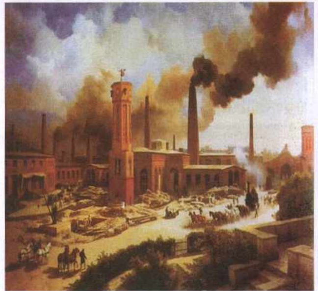
Smoke from several factories polluting the air during the Industrial Revolution
