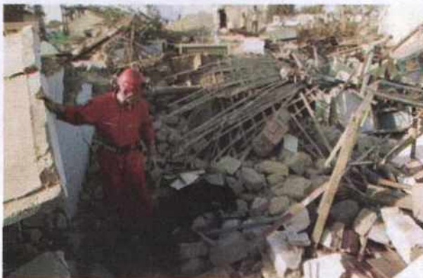
Widespread destruction after the earthquake in Gujarat
