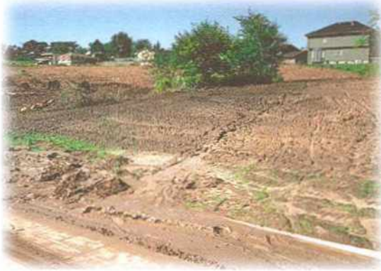
Fig. 6.2 Soil erosion caused by water
