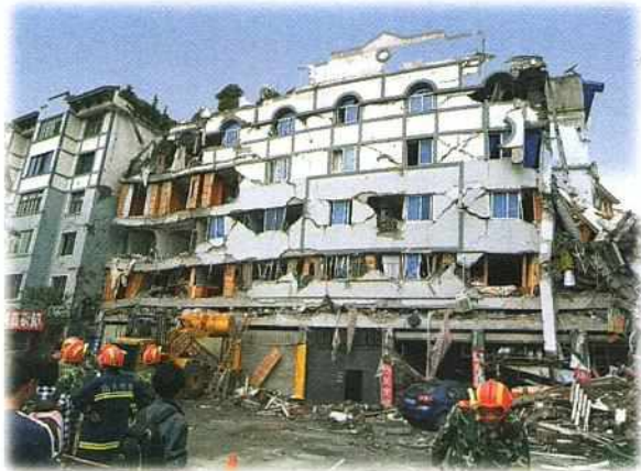
Fig. 14.1 A building collapsed during an earthquake
