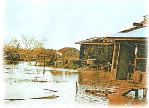
Fig. 14.5 Destruction caused by tidal waves
