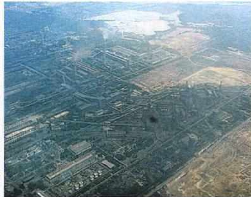
An aerial view of the Visakhapatnam Steel Plant
