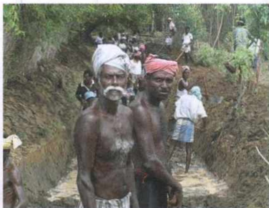
Building a road—rural employment generated under the Sampoorna Grameen Rozgar Yojana
