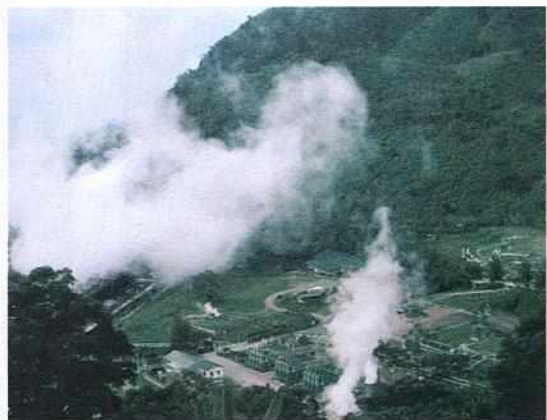
Puhagan Geothermal plant, Philippines
