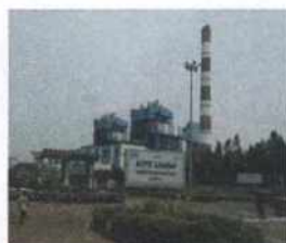
NTPC plant at Simhadri
