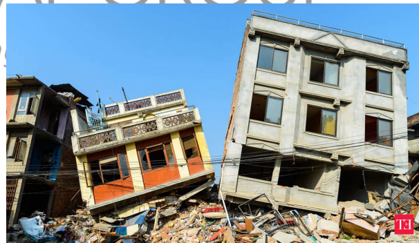
Buildings are collapsed during an earthquake
