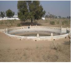
4 The **tankas** are part of the well-developed rooftop rainwater harvesting system.
